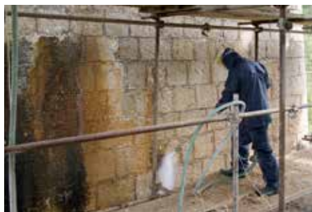
Cleaning building scaffolding
